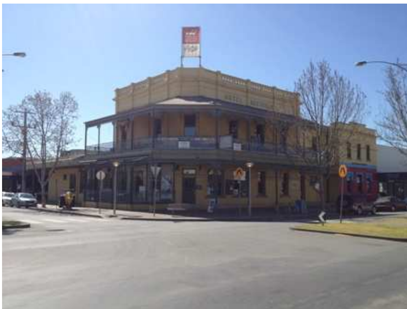
73-83 Fryers Street, Shepparton - Hotel Australia
