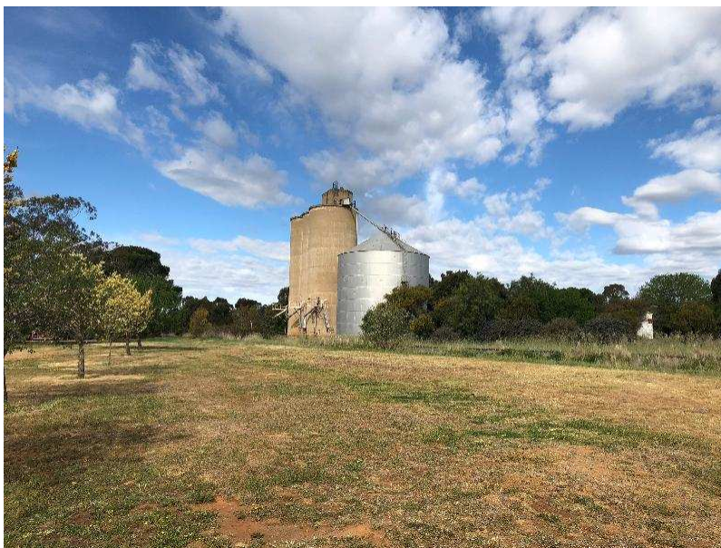
7 Baldock Street, Dookie (Silos)
