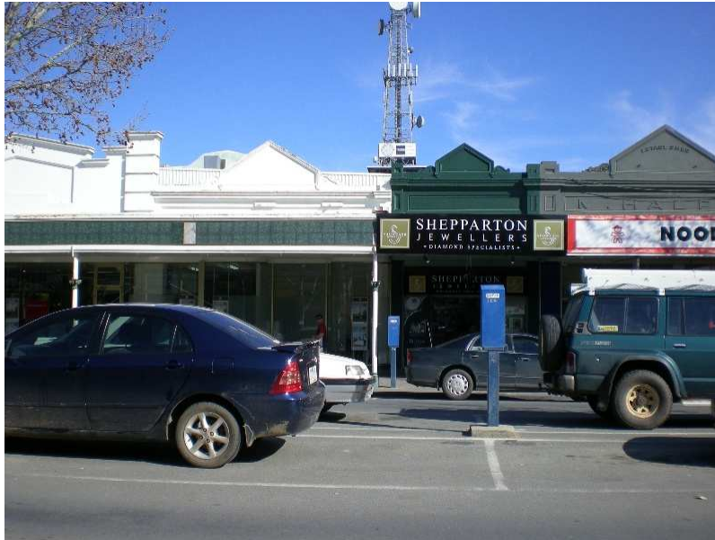
54-56 Fryers Street, Shepparton
