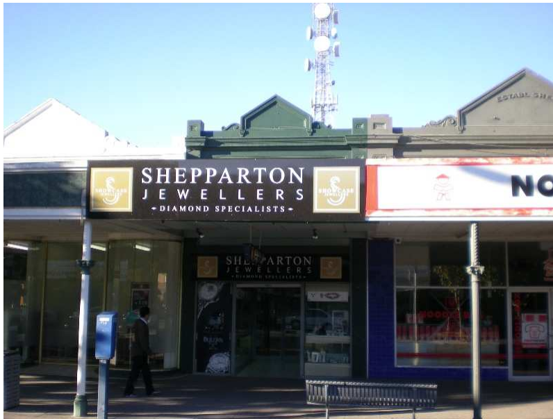
52 Fryers Street, Shepparton
