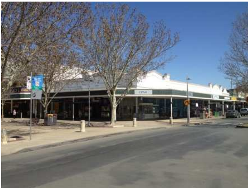
52-62 Fryers, 174-198 Maude and 285-289 Wyndham Streets - Fairleys Building
