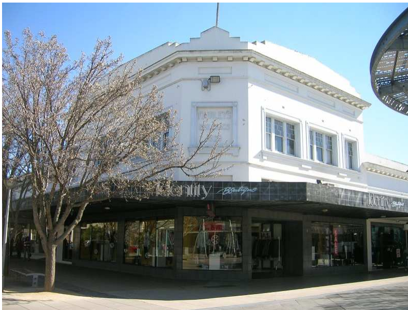
13-23 Fraser and 200-210 Maude Streets, Shepparton - Fairleys Building
