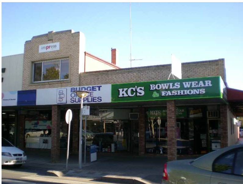
97-101 Fryers Street, Shepparton
