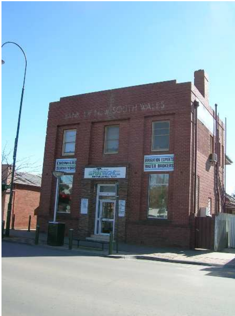
139 Hogan Street Tatura former Bank of NSW
