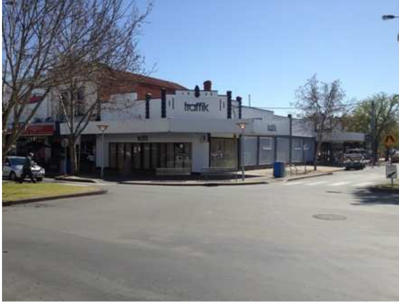
69-71 Fryers Street, Shepparton
