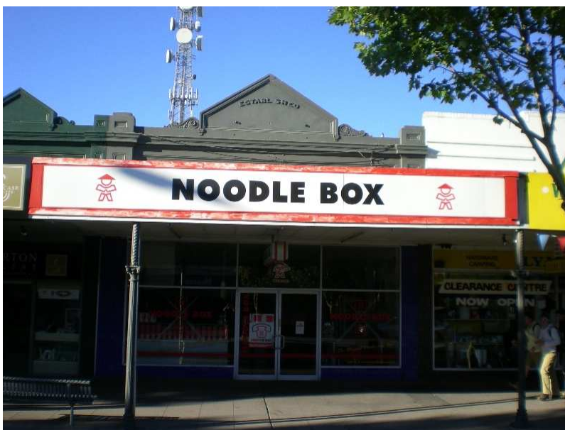
50 Fryers Street, Shepparton
