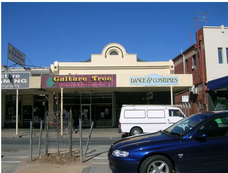
86-88 Fryers Street, Shepparton
